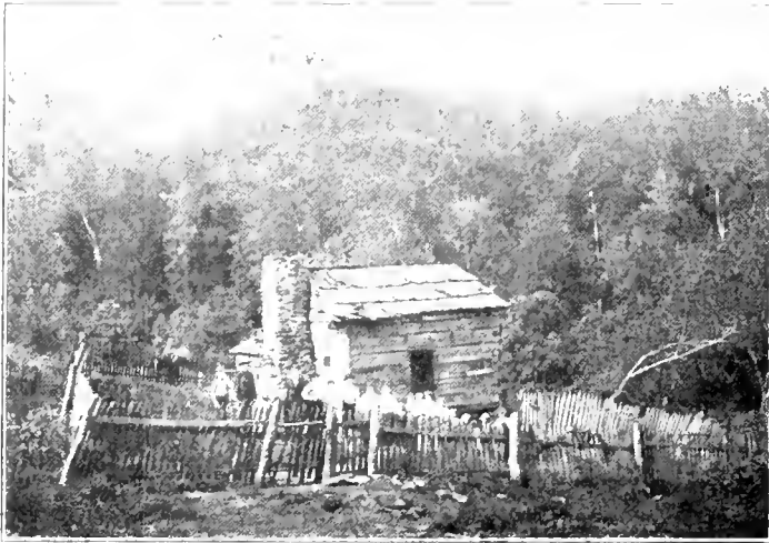
TYPICAL CABIN OF MOUNTAINEER, WEST VIRGINIA
